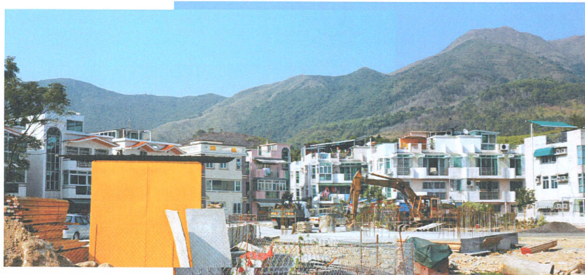
LCA 4 - VILLAGES : SOIL DUMPING AND CONSTRUCTION ACTIVITIES ADJACENT DEVELOPMENTS
