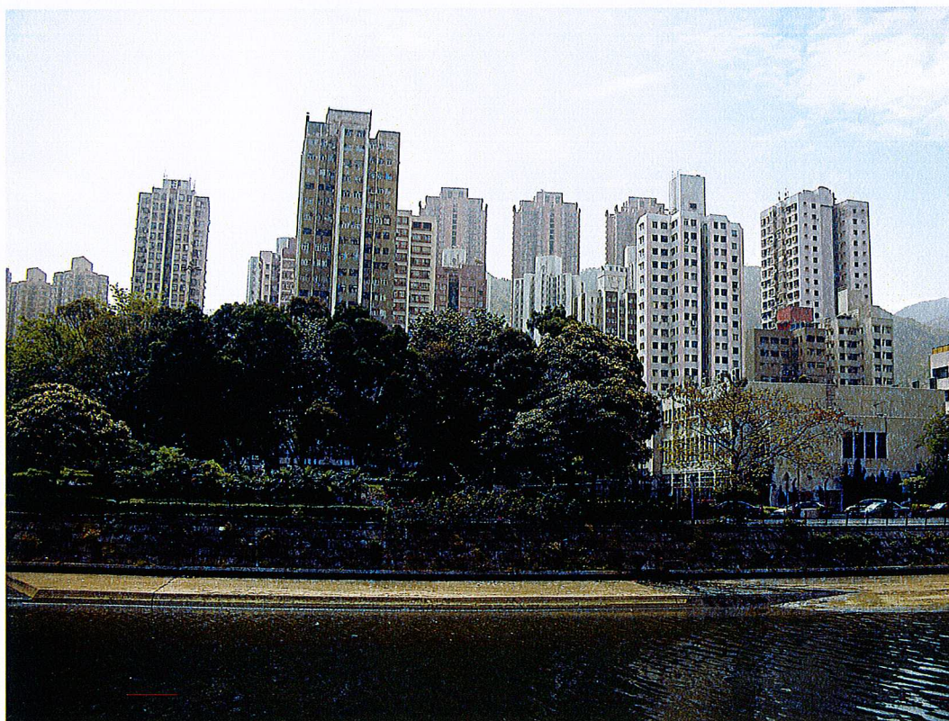
Photo 2: Residential Buildings near Tuen Mun Road
