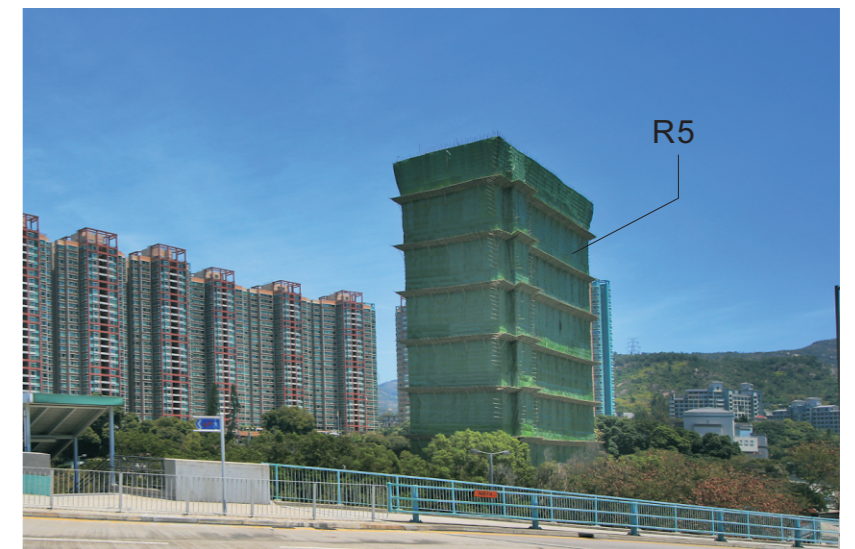
R5 Tuen Mun Fire Services (R&F) Married Quarters
