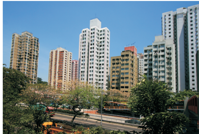
R2A Kam Fat Building, Yan Oi Building, Lam Kwong Building and Kam Men Mansion
