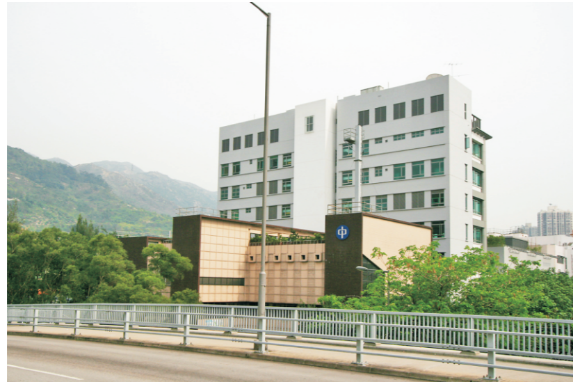
GIC6 Tuen Mun Church, Tuen Mun Tseng Choi Street Joint-user Complex, and Electric Sub-station
