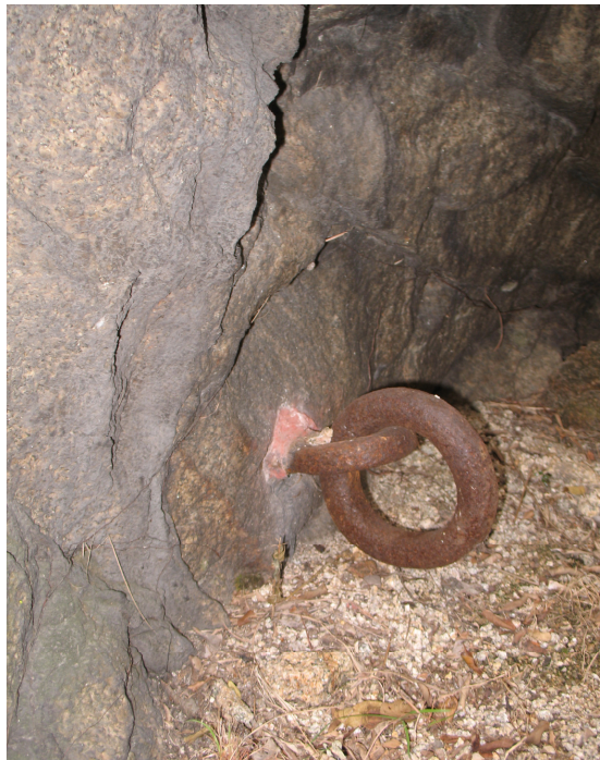
View of metal ring used for transporting of guns and equipment to the old West Battery 用作運送槍炮及裝備往前西炮台的鐵環
