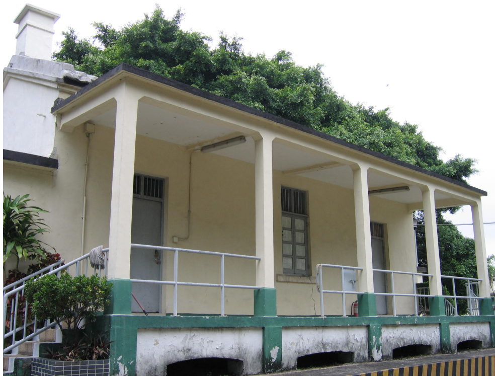
Front view of Block 29 (Old West Battery) 第二十九座(舊西炮台)
