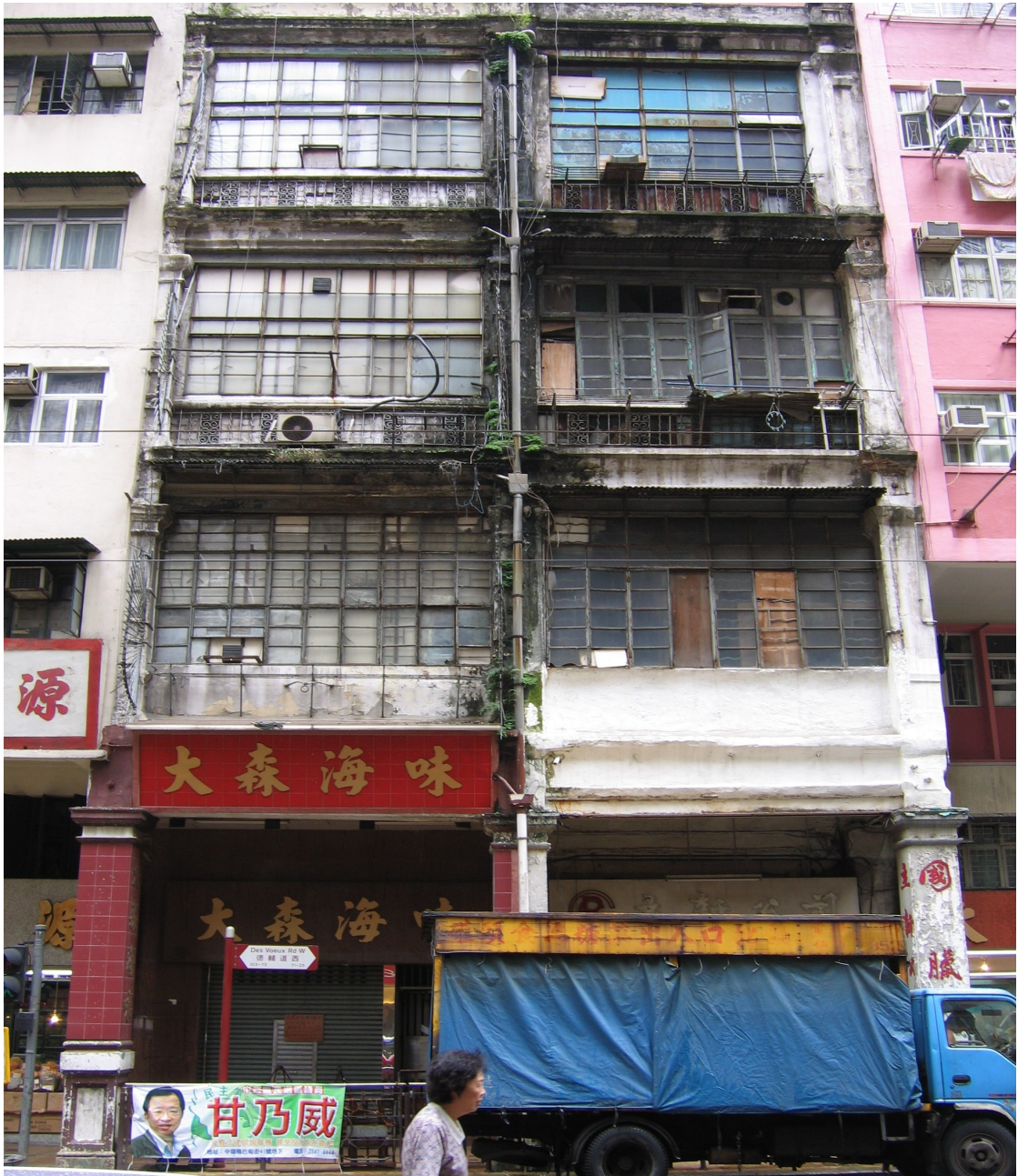
View of the two shophouses at 67 and 69 Des Veux Road (HATS – 04) 中環德輔道西 67, 69 號
