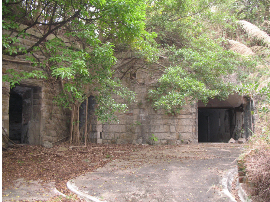
View of the ruins of magazines associated with the former West Battery 前西炮台軍火庫遺址
