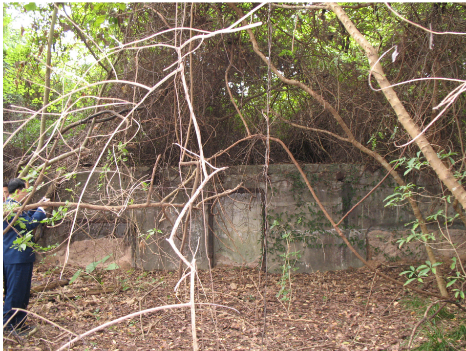
View of magazines associated with the old Central Battery 中炮台舊軍火庫遺址
