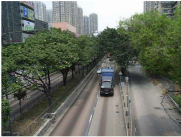
Photo A09 LR5 Street trees along Tuen Mun Road west of Waldorf Garden and CMA Choi Cheung Kok Prevocational School
