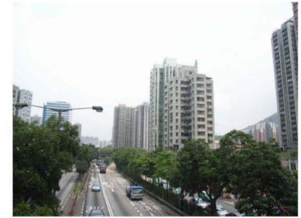
Photo A08 LR4 Street trees along Tuen Mun Road west of Chi Lok Fa Yuen and east of On Ting Estate
