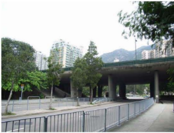
Photo A05 LR3 Street trees along Castle Peak Road - Castle Peak Bay
