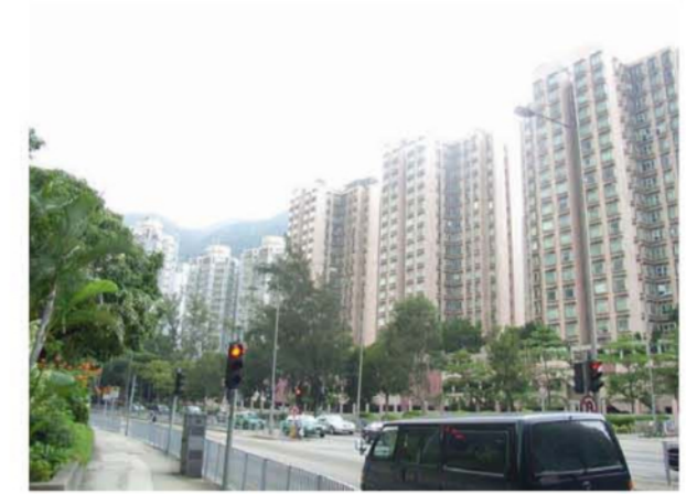
Photo A04 LR3 Street trees along Castle Peak Road - Castle Peak Bay Garden
