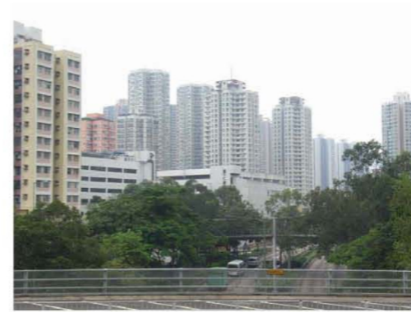
Photo A11 LR7 Street trees along Tuen Mun Road east of Yan Oi Tong
