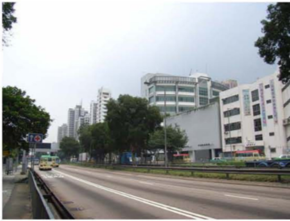
Photo C05 GIC1 Tuen Mun Church and Tuen Mun Tseng Choi Street Joint-user Complex
