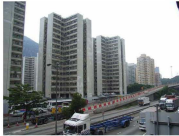
Photo C18 R4 Residential Area along Tsing Hoi Circuit
