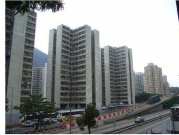
Photo C27 T1 Tuen Mun Road – Vehicular and Pedestrian
