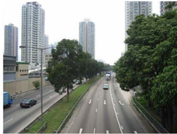
Photo C30 T1 Tuen Mun Road – Vehicular and Pedestrian
