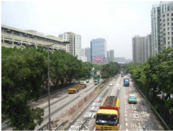
Photo C29 T1 Tuen Mun Road – Vehicular and Pedestrian
