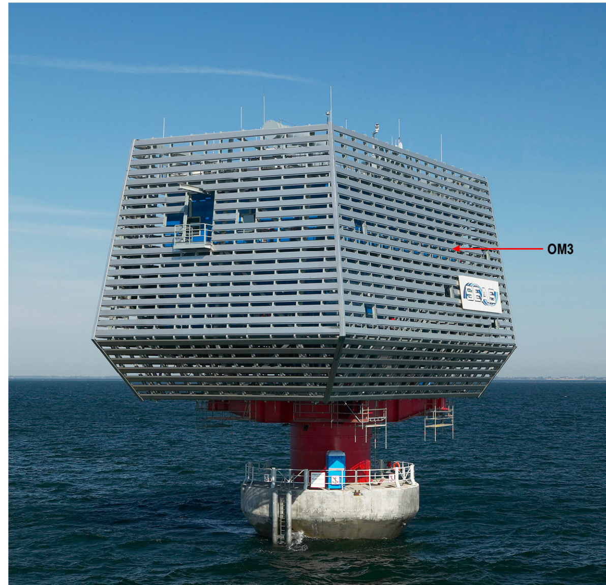
TYPICAL TRANSFORMER STATION DESIGN AND FINISH TREATMENT
