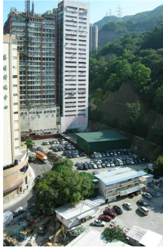
Kwai Chung Ventilation Building (KWV)
