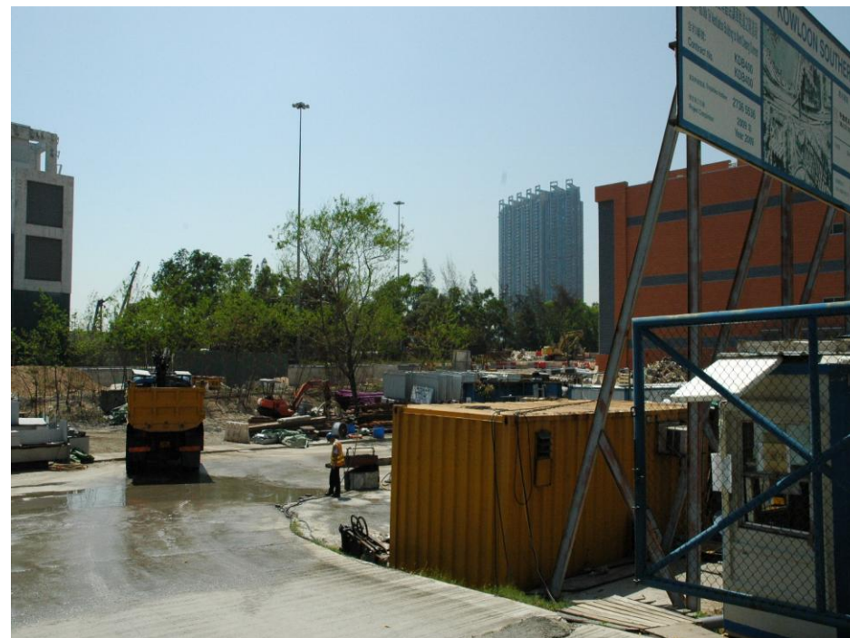
Works area near MKV
