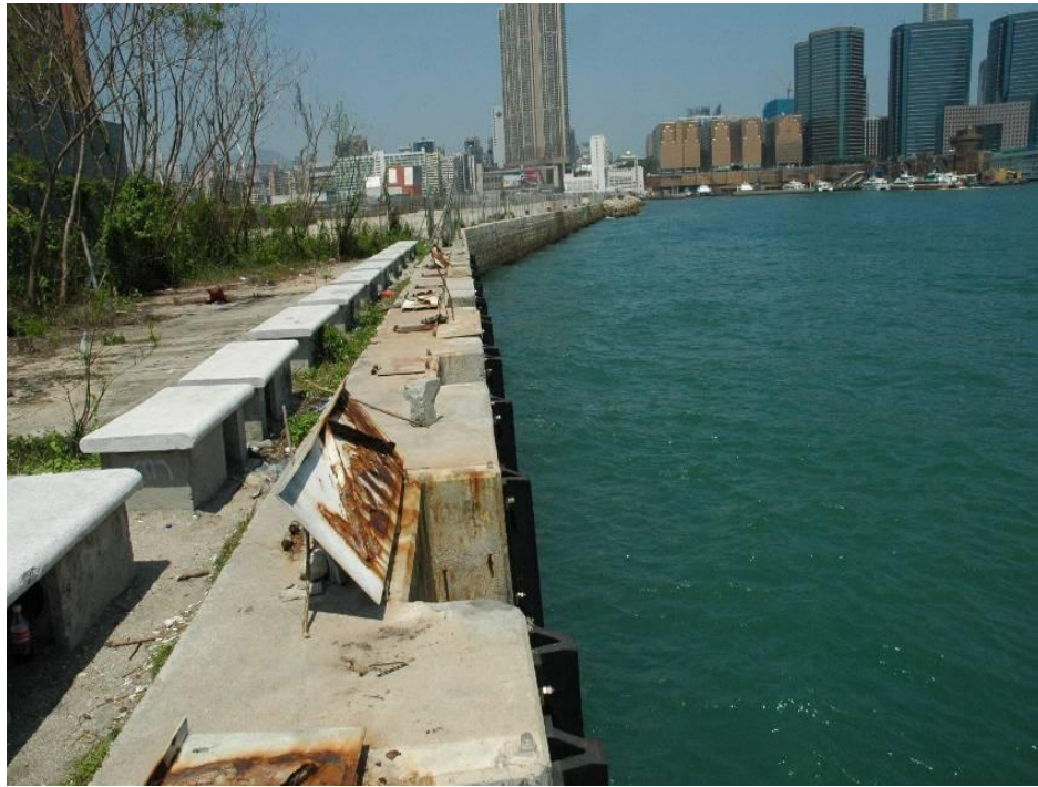
West Kowloon Barging Point (WKB)
