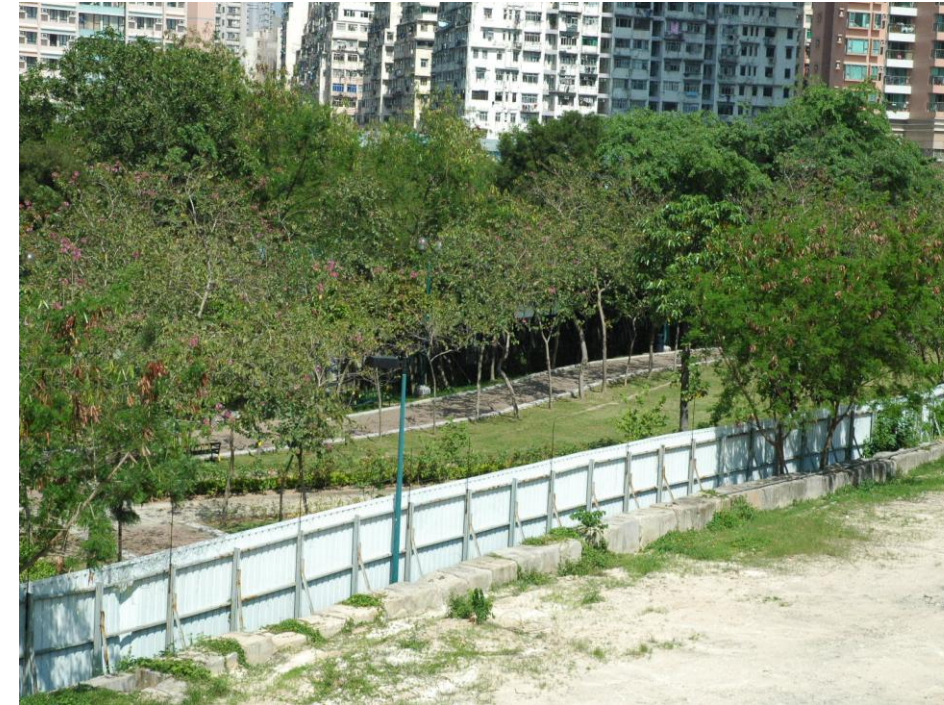
Works areas near NCV
