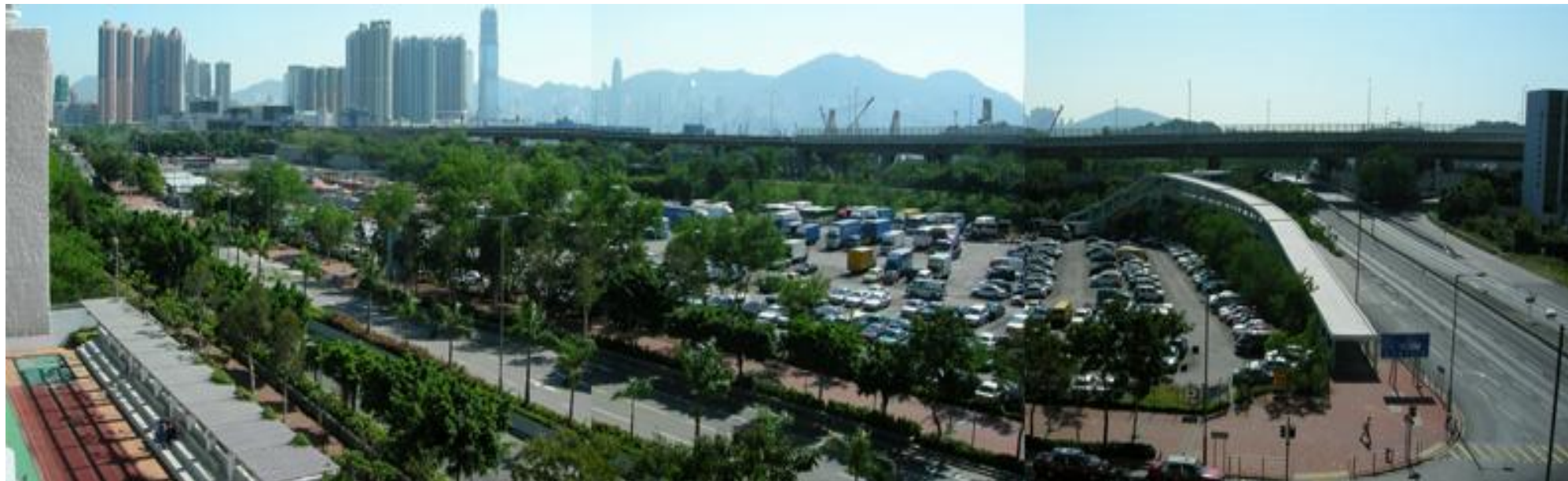
Nam Cheong Ventilation Building (KCV)
