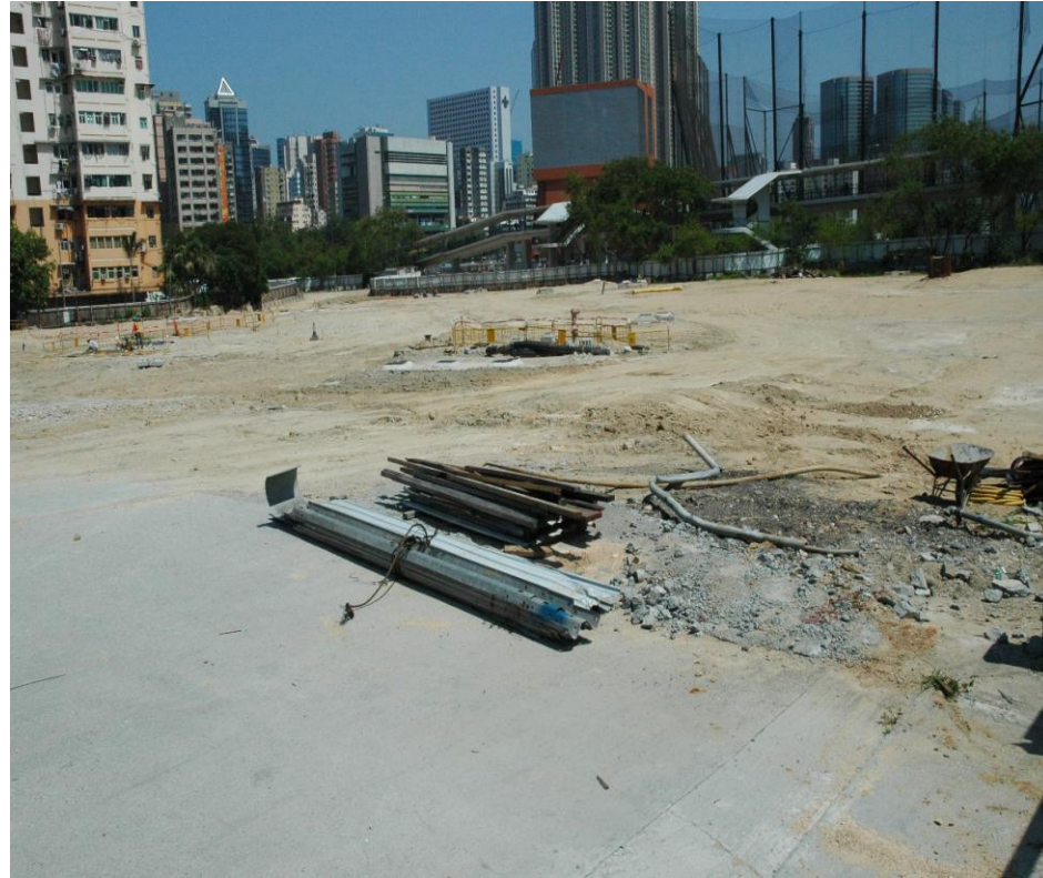
Mong Kok West Ventilation Building (MKV)
