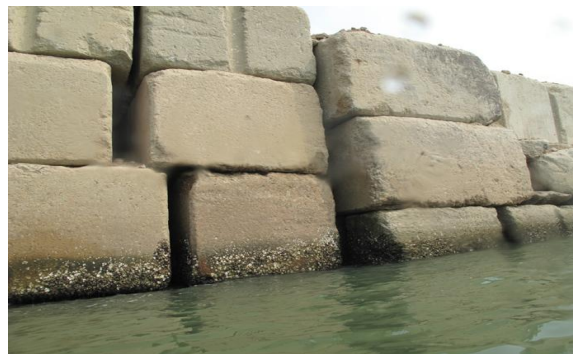
Artificial Vertical Seawall
