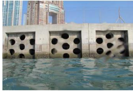
Artificial Vertical Seawall
