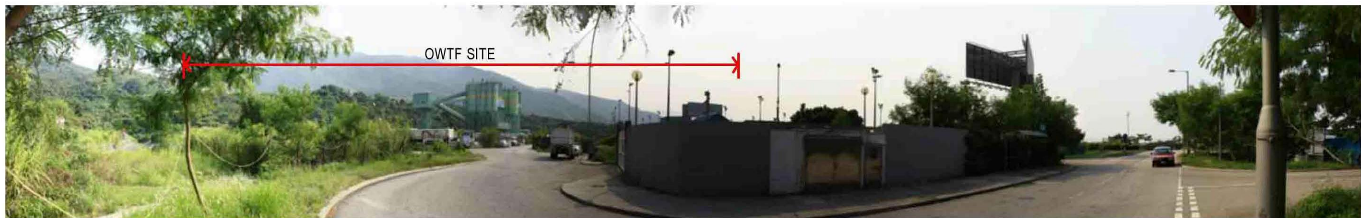
VSR2 VIEW ANGLE "B" View from Outside the Bus Depots
