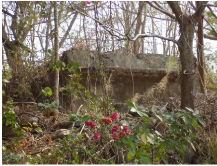
Plate 34a View of ruined structure associated with the former Aberdeen Battery
