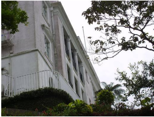
Plate 41b Front View of House No. 33 Magazine Gap Road
