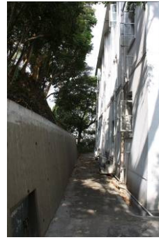
Plate 10b Southwest elevation of the Old Victoria Barracks Robert's Block
