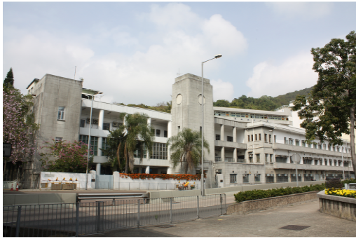
Plate 5c View of the façade of the Aberdeen Technical School
