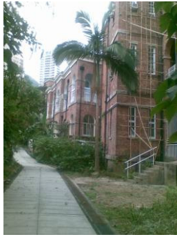
Plate 7c View of the rear elevation of the Former British Military Hospital
