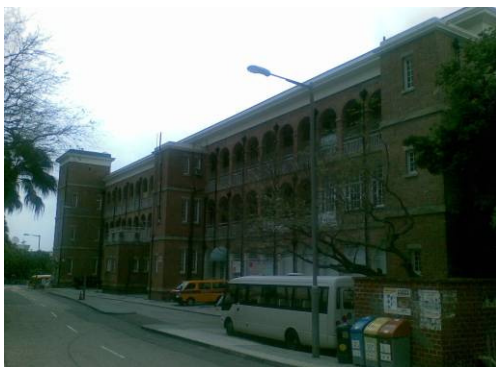
Plate 7a View of the façade of the Main Block of the Former British Military Hospital
