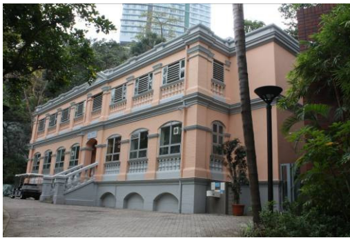
Plate 11a Northwest elevation of the Old Victoria Barracks Wavell Block
