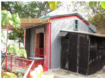
Plate 32b Northwest elevation of the Tai Wong Temple on Ap Lei Chau
