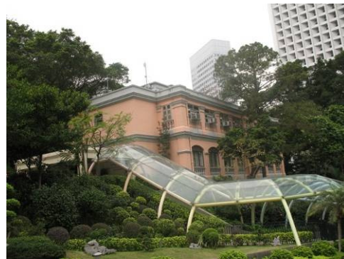
Plate 12 View of the south elevation of Rawlinson House
