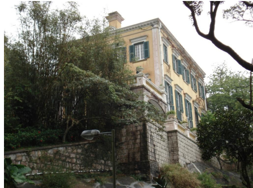
Plate 43a Side View of House No. 15 Middle Gap Road
