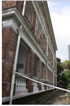
Plate 10a Northeast elevation of the Old Victoria Barracks Robert's Block
