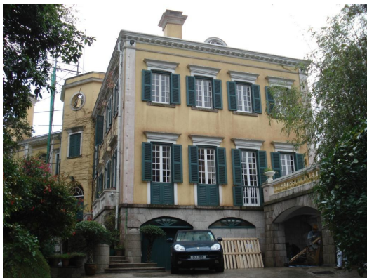
Plate 43b Front View of House No. 15 Middle Gap Road
