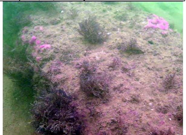
Spot 4 (ES4) – Vertical sea wall with waste tyres and wood at bottom
