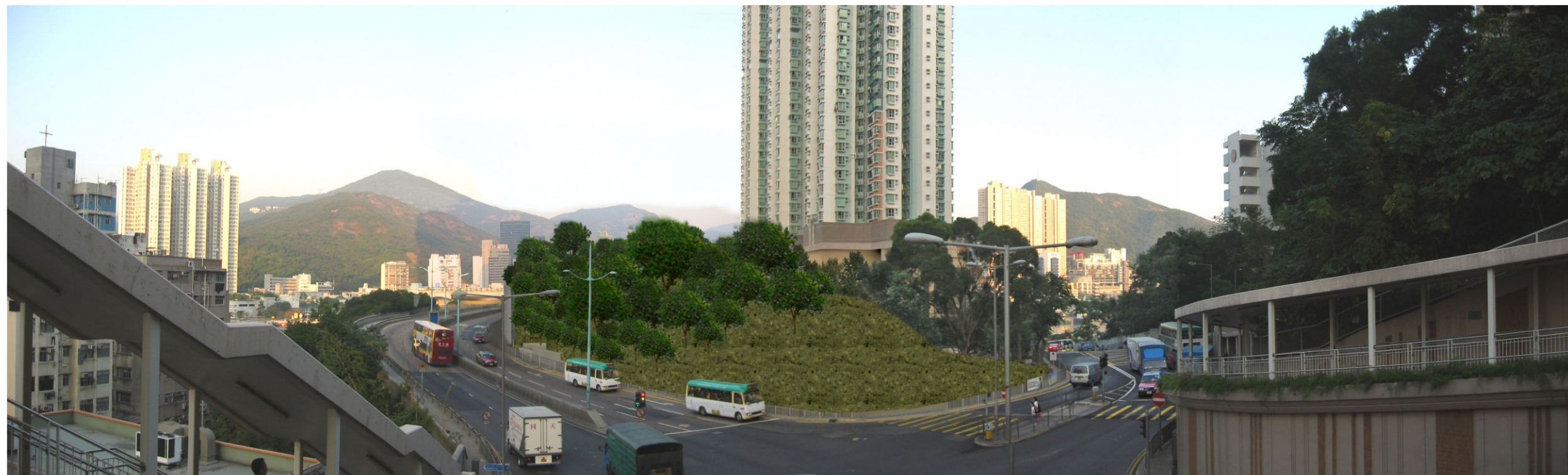
Year 10 of Operation Phase with landscape mitigation measures fully established
