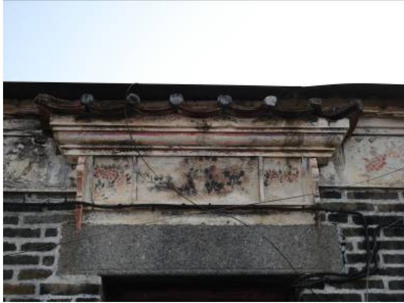
Decoration above lintel of No. 48 Tsung Yuen Ha
