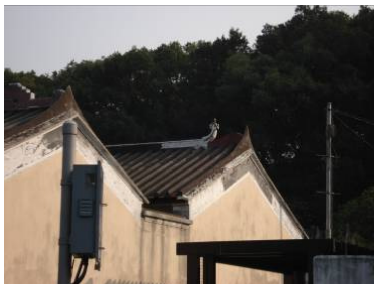
Roof Ridge Decoration
