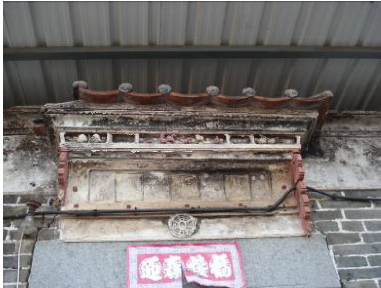
Decoration above lintel of No. 50 Tsung Yuen Ha
