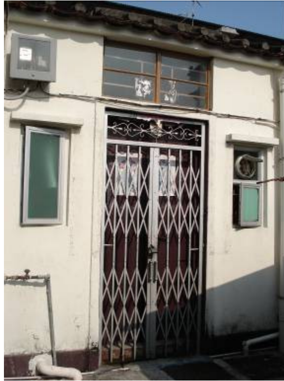
Front View of No. 23B Kan Tau Wai
