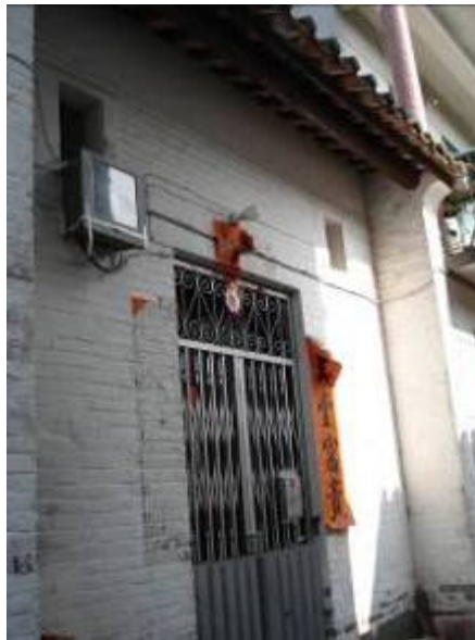
Front door and tile roof above
