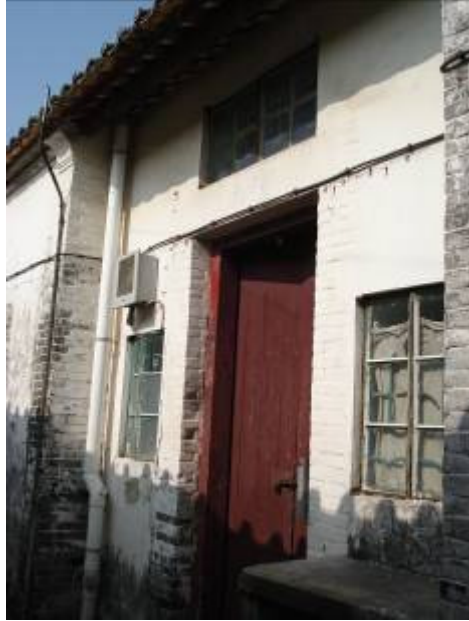
Front View (Doors and Windows) of No. 16 Kan Tau Wai
