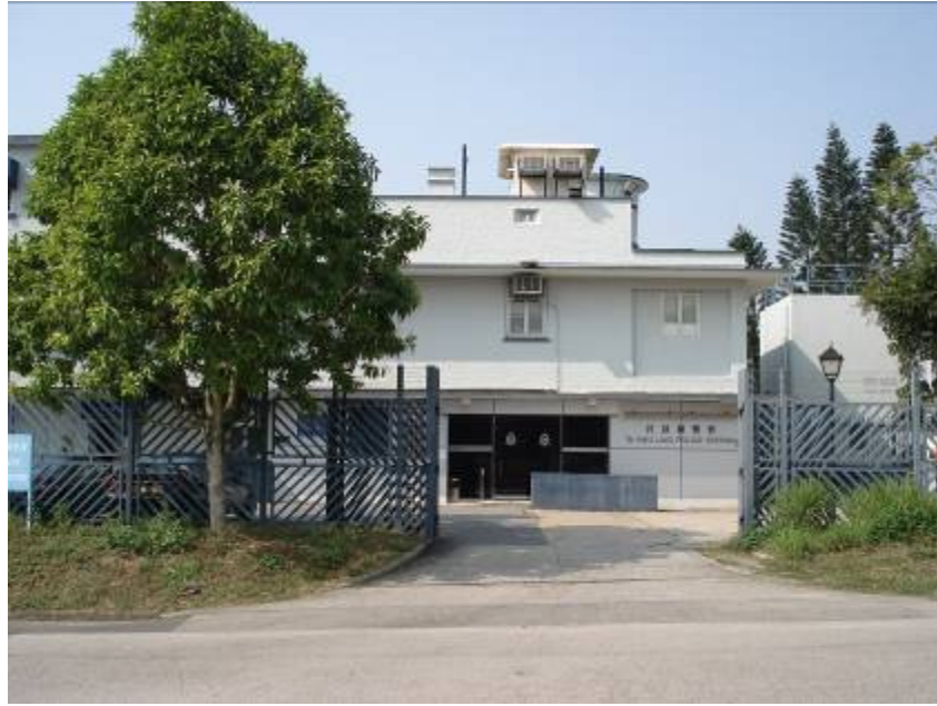
General View of Front Gate
