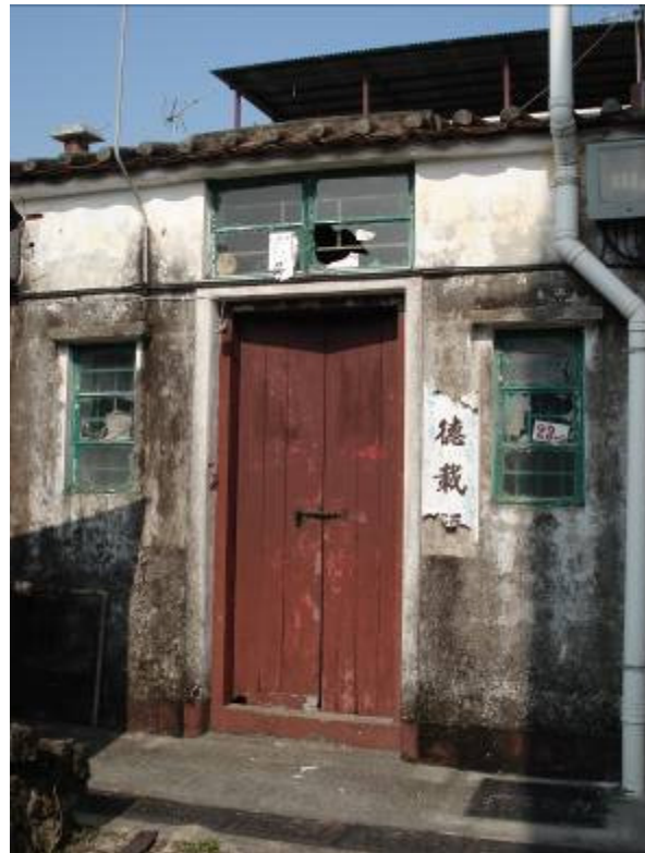
Front View of No. 23C Kan Tau Wai
