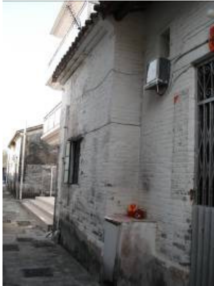
Another angle of front view
