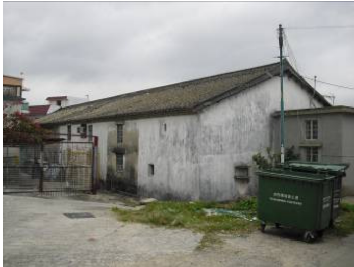
General Back View of Nos. 51-56 Ping Yeung
