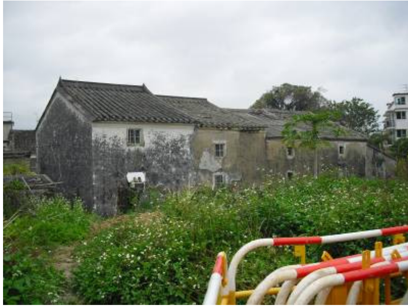
Back View of Nos. 1-3 Ping Yeung (from right to left)
