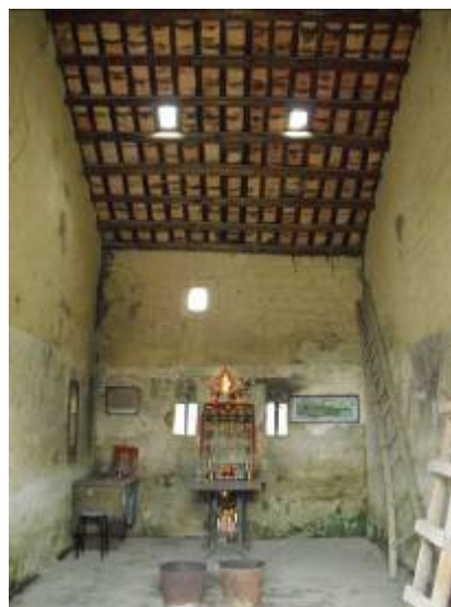
Interior View of No. 54 Ping Yeung
