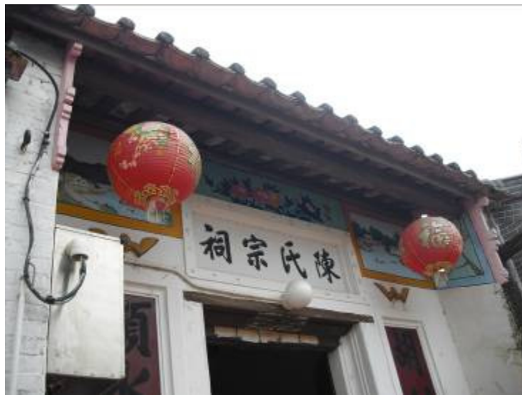
Tile roof and external decorations
