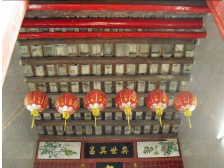
Tile roof and wooden beams
