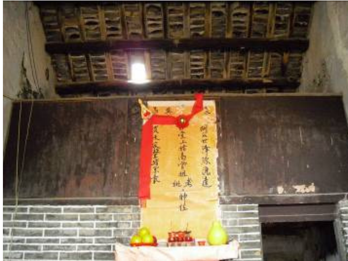
Tile roof and wooden beams
