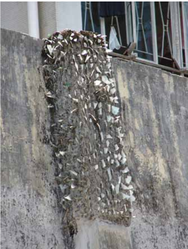
Shards of glass embedded in cement at the tops of the buttresses along the south wall
