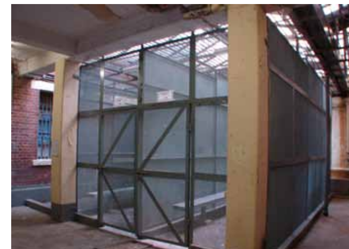
Figure 12 - Cells on the ground floor which have been constructed within the lightwell
