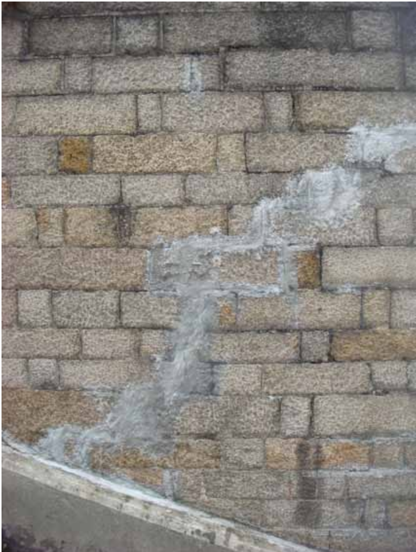
A poor quality repair to stonework in EX08-A
