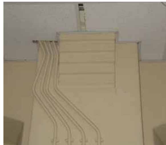
Figure 9 - Brick corbel probably added to support a new concrete floor on the new third floor
