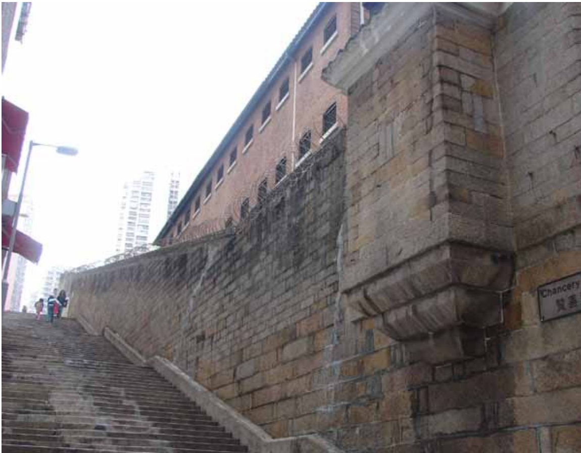
Figure 2 - The projecting 'lookout' with granite corbel support on the south side
