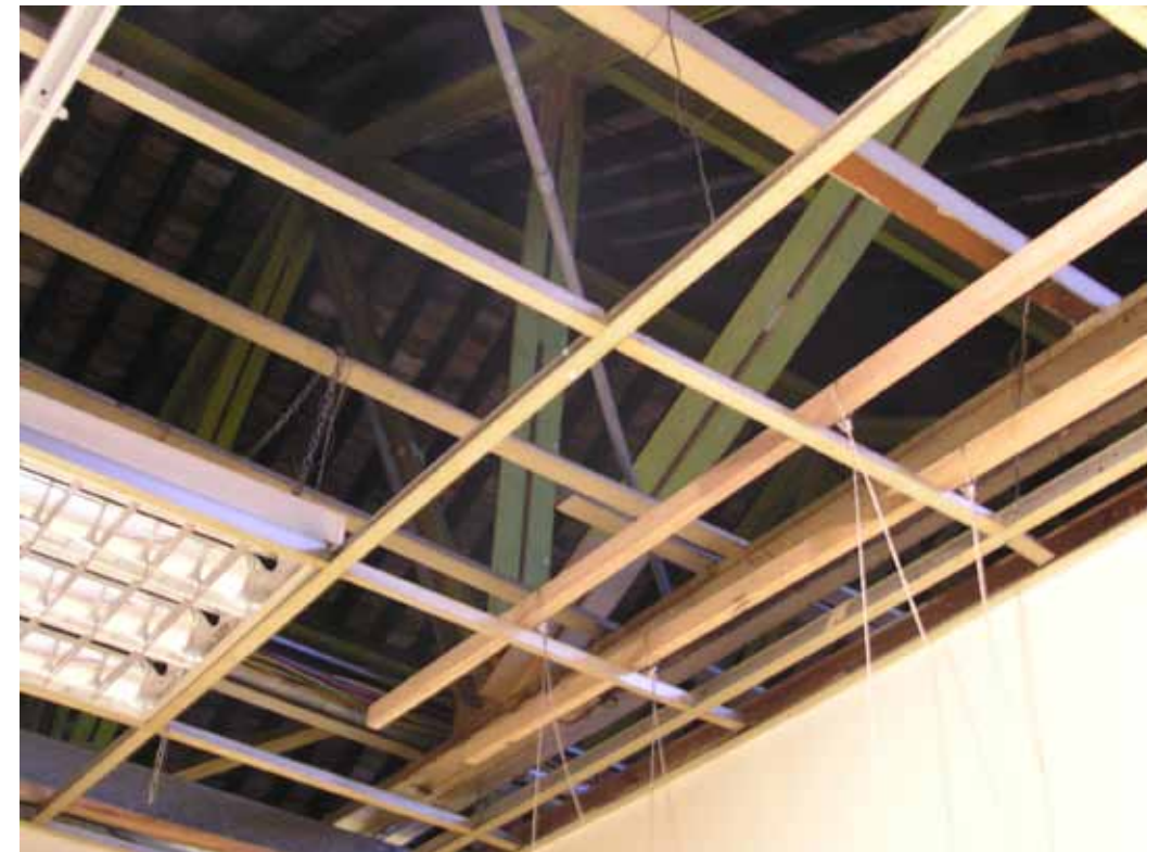
Figure 15 - Steel truss roof structure. The lower grid is the modern inserted ceiling. The original ceiling is above the rafters.
