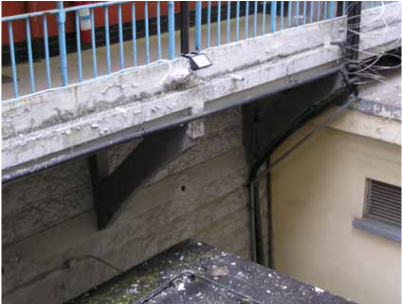
Figure 4 - Supporting brackets for the balconies
