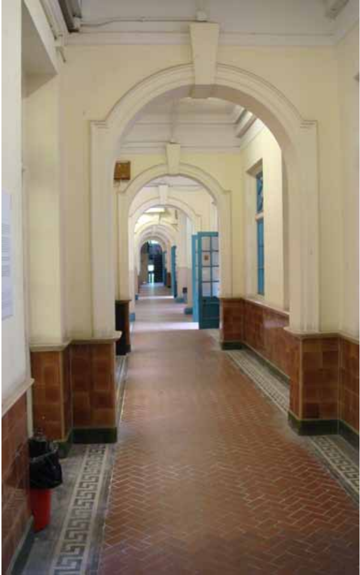
Figure 8 - The ground floor corridor with decorative keystone arches, Canton tile floor with Greek key border and glazed tiled dado
