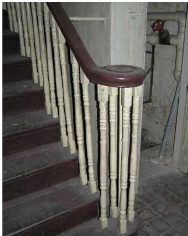
Figure 9 - Main staircase balustrade and moulded timber handrail, as viewed on the ground floor.
