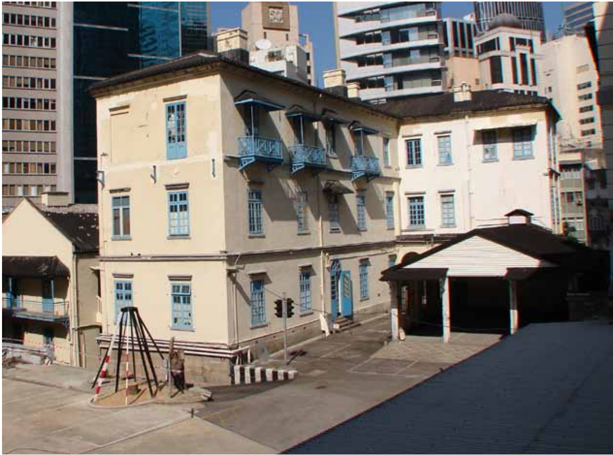
Figure 2 - Southwest elevation; note the missing balcony on the west end, second floor
