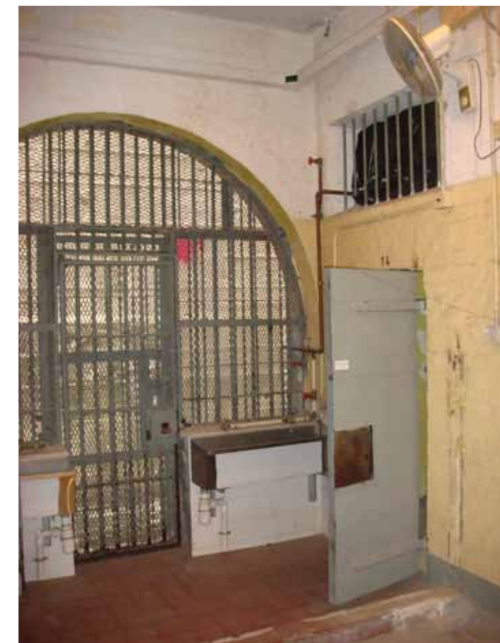
Figure 9 - The ground floor archway at the west end of the building. Note the later door on one of the cells and the sinks installed at an unknown date.
