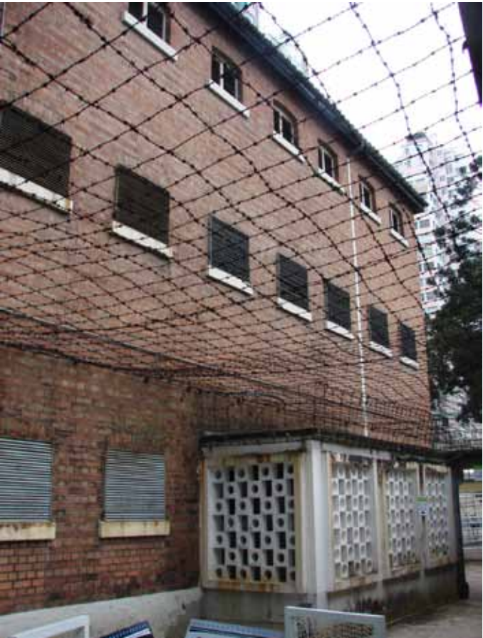
Figure 4 - The entrance to the Laundry, a perforated concrete surround over the stairs; this is adjacent to the north side of E Hall
