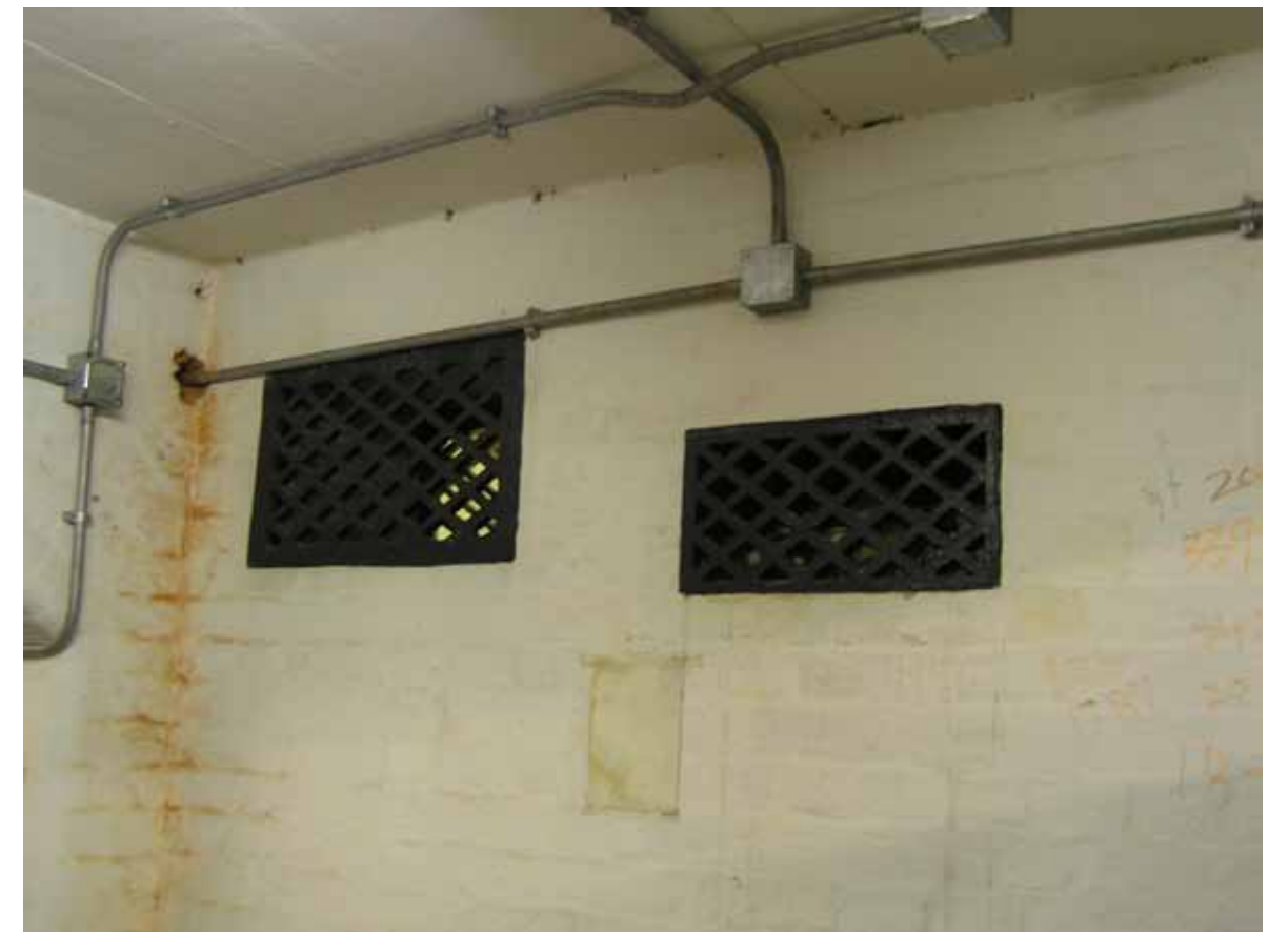
Figure 13 - Lattice ventilation grilles in the basement
