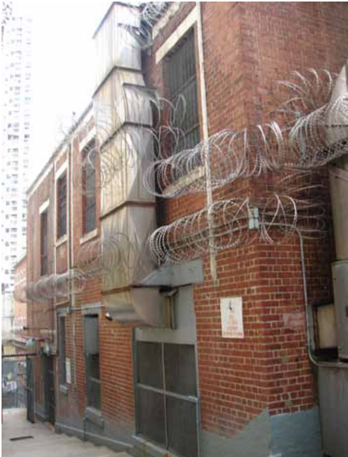
Figure 1 - Exterior view of the south elevation, showing a large exhaust duct from a kitchen window
