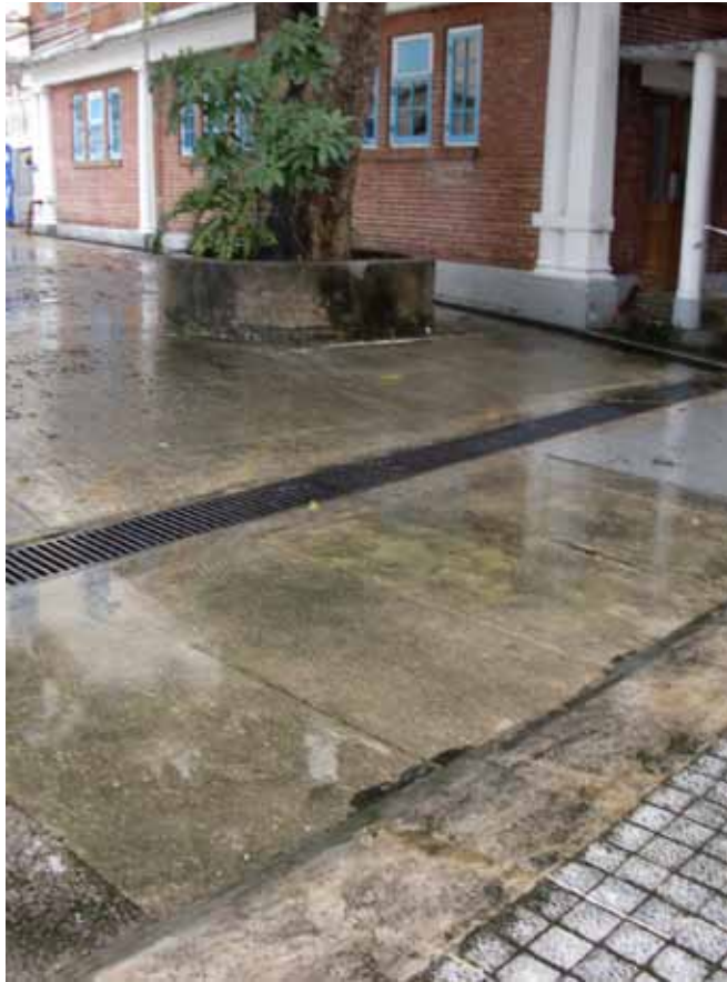
Paving slabs to the south of Building 01, adjacent to which are cast iron grilles for drainage and some areas of small concrete tiles
