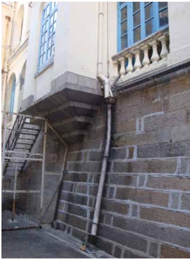
Figure 6 - Granite corbel supporting one of the north projecting bays. The other is in need of urgent repair.
