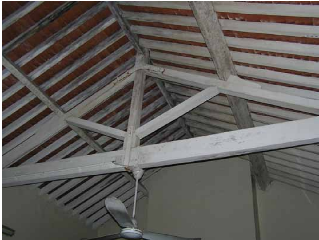
Figure 15 - Timber frame roof structure visible on the first floor of the southwest extension
