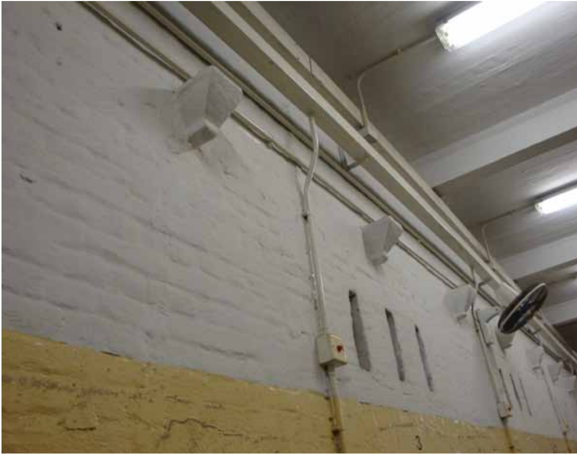
Figure 7 - Corbels in the west wing first floor which indicate the original level of the ceiling
