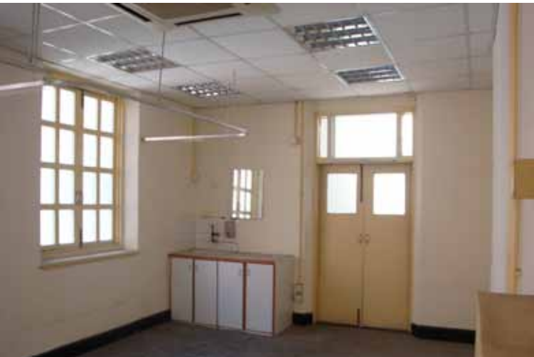
Figure 5 - Typical interior space, with later suspended ceilings and replacement double doors. The fanlight has been altered to accommodate air-conditioning.
