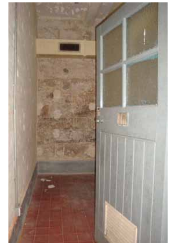
Figure 13 - Timber batten door at ground floor level
