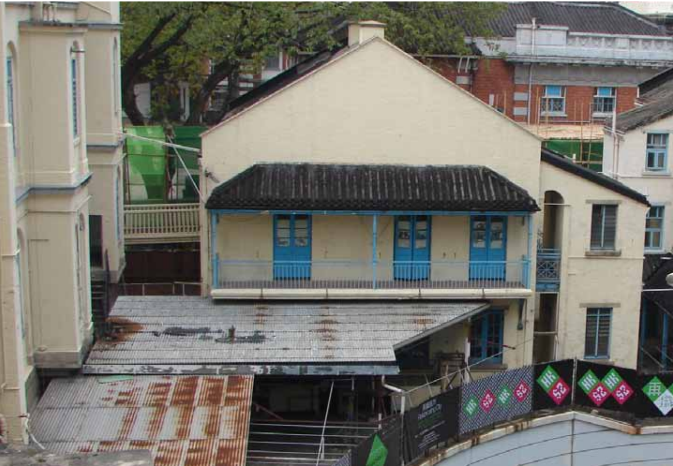
Figure 1 - East elevation of the building. The corrugated iron coverings have been partially removed since this photograph was taken.
