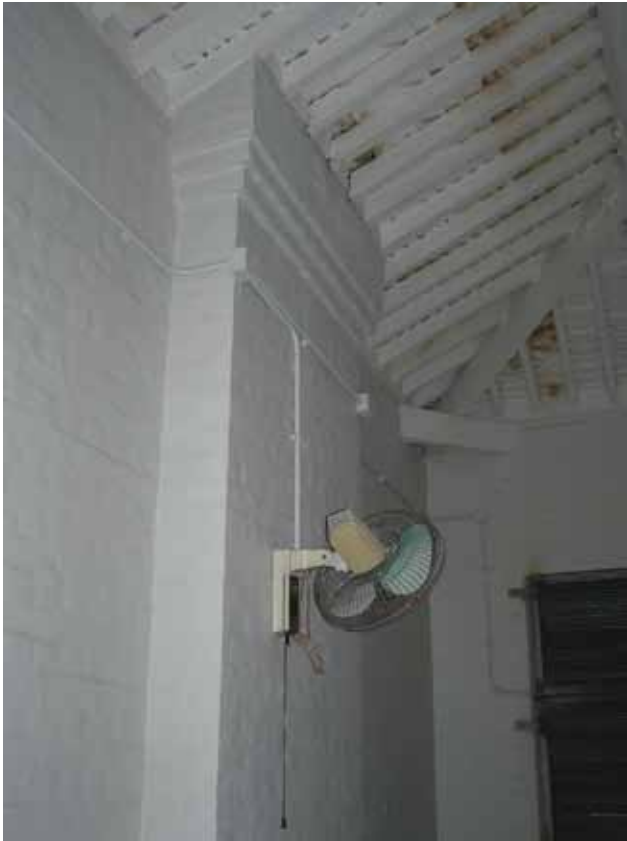
Figure 5 - First floor brick chimney breast
