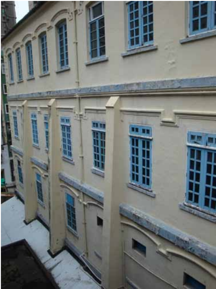
Figure 3 - Partial view of the south elevation showing blocked windows on the ground floor, and buttresses added c.1906
