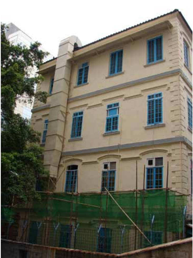
Figure 4 - West elevation showing large ductwork for one of the modern kitchens and third floor corrugated metal sunshade
