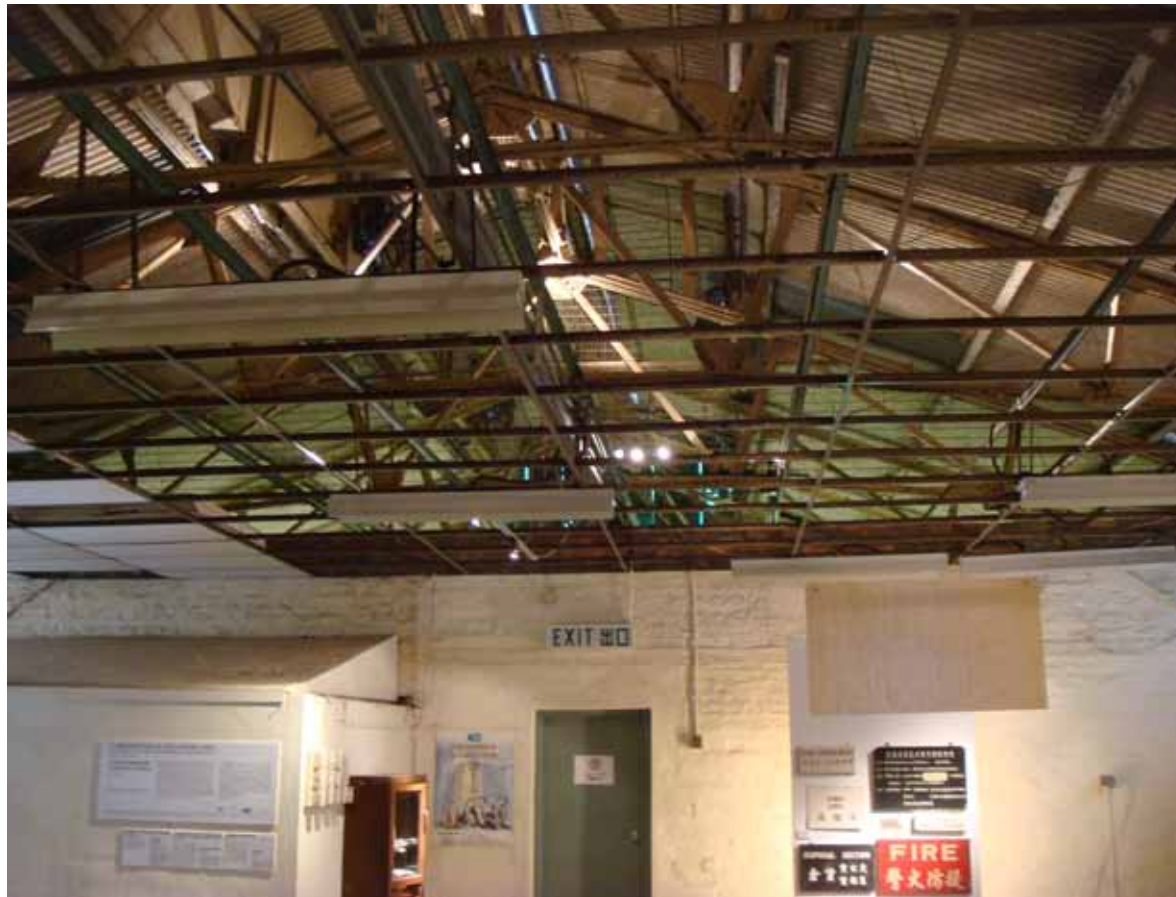
Figure 5 - Interior of the covered yard showing the steel frame roof structure
