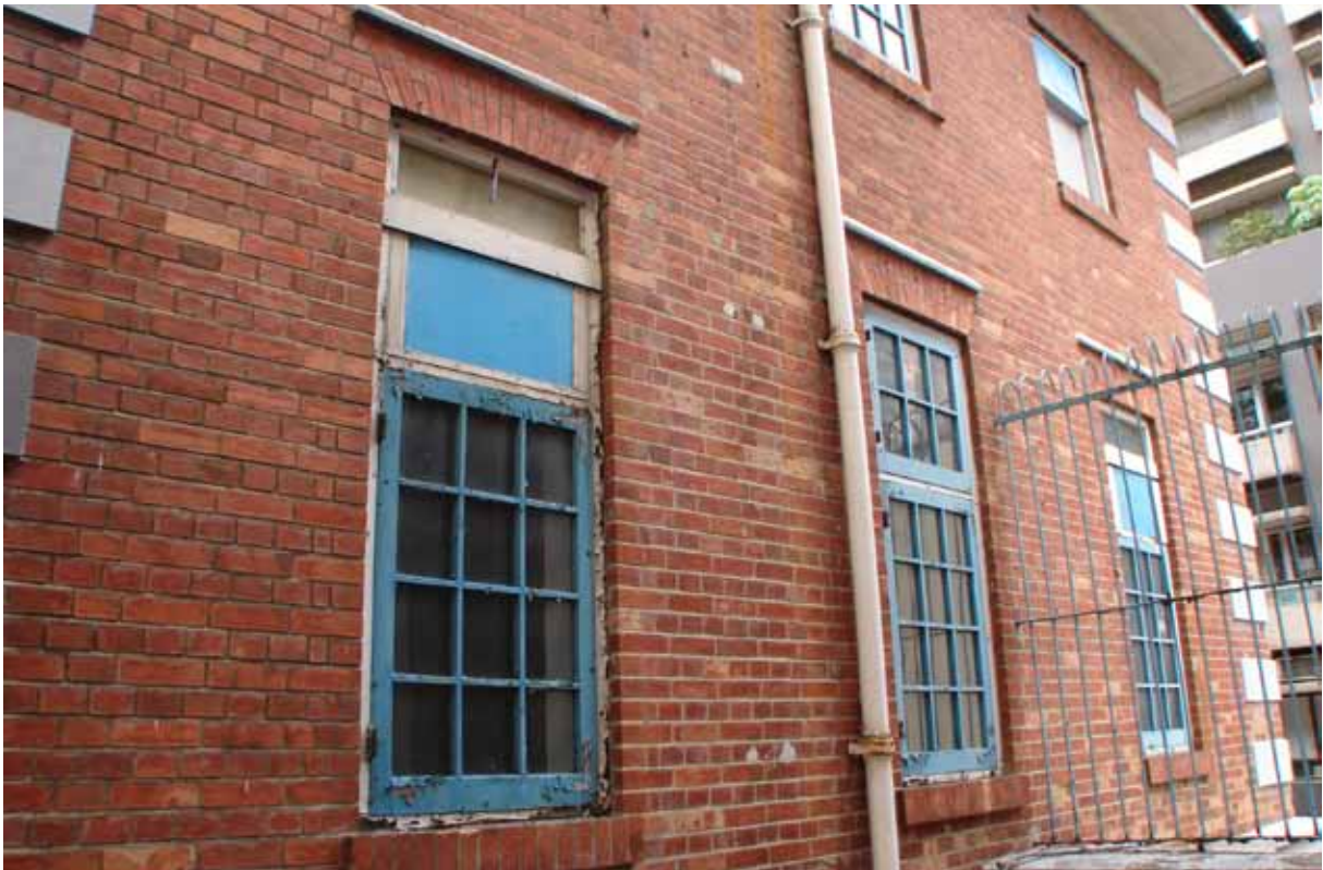
Figure 3 - Windows on the south elevation. The ground floor central window has the original/early casement with fanlight casement above, while those either side have been altered to accommodate air conditioning units.
