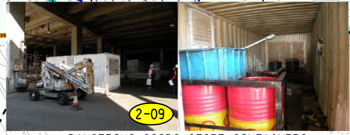
DANGEROUS GOODS STORE CONTAINERS (APPROXIMATELY 20 m 2 )
