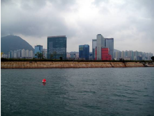
KT3 - Artificial seawall
