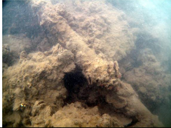
KT1 - Trash plastic pipes
