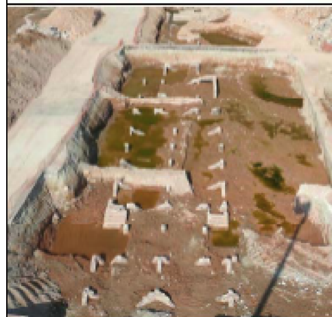
VIEW C SUPPORTING PILLARS OF FORMER KOWLOON CITY PIER
