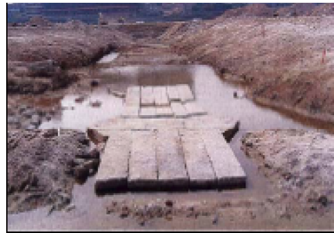
VIEW A LUNG TSUN STONE BRIDGE PIER
