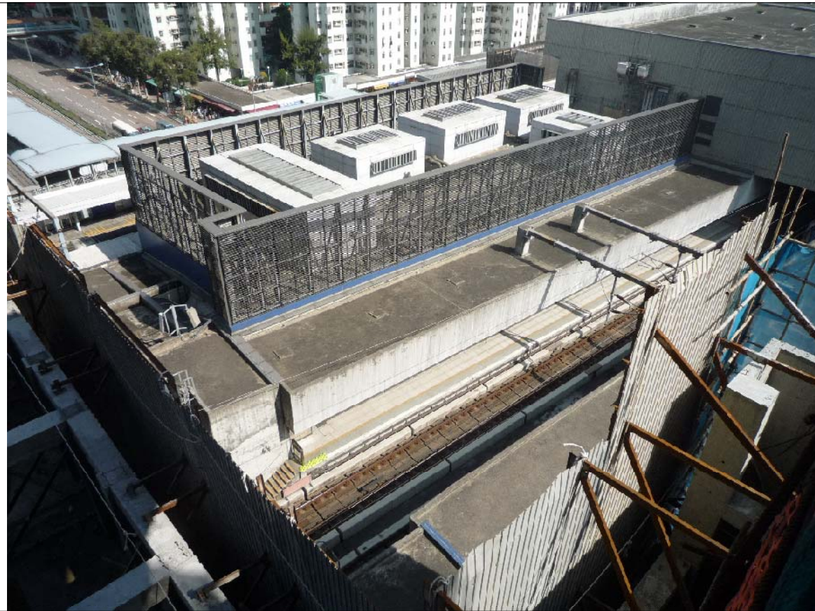
PM2 - EXISTING VIEW
