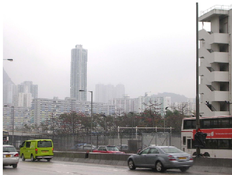
DIH & KAT - LR 3.7 - TREES AT JUNCTION OF EASTERN ROAD AND CONCORDE ROAD
