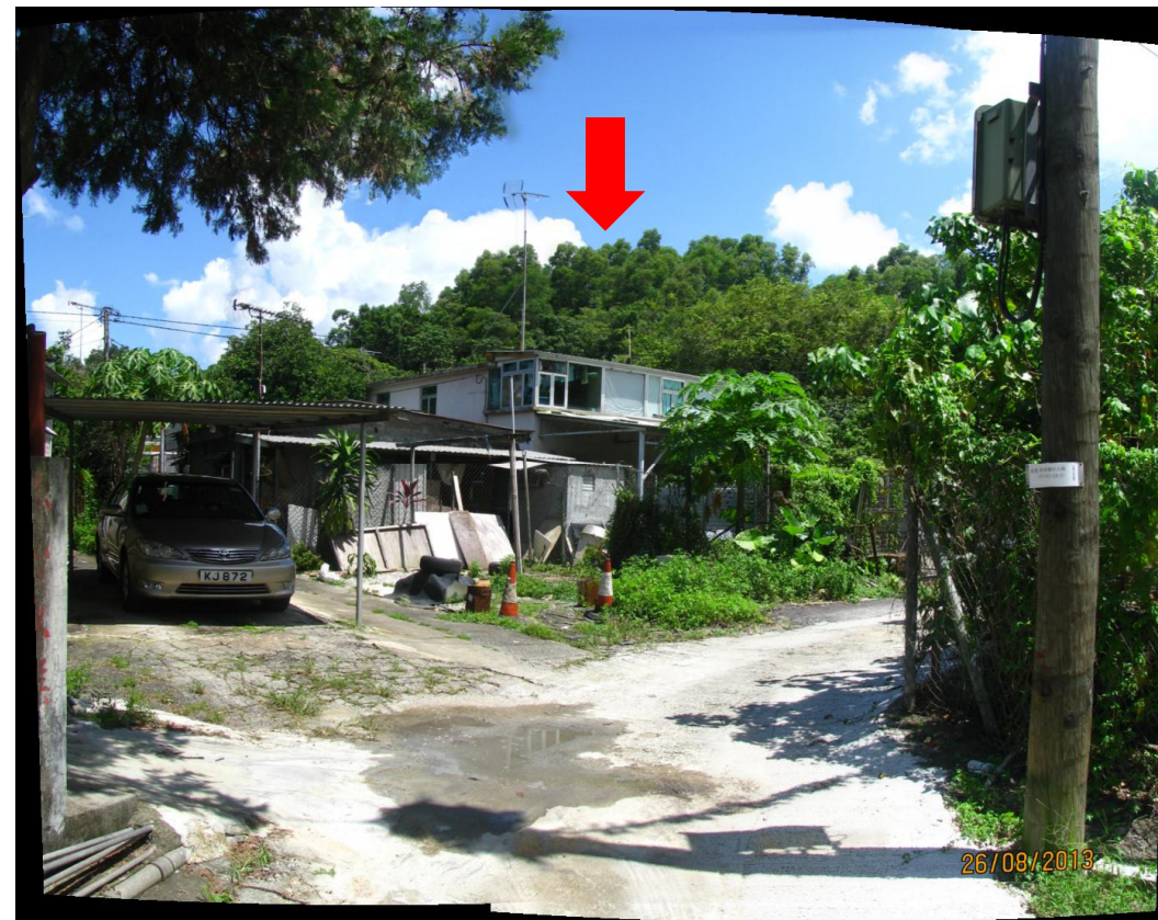
VSR3.1 – View from Village from the Northwest
