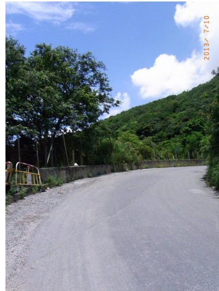
Plate 2. Developed Area within the Study Area comprises only the existing construction site to the west of Anderson Road, Anderson Road (shown in Plate 2) and southern section of Po Lam Road.
