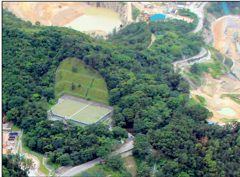
LR7.1 Utilities Landscape at Rural Development Area
