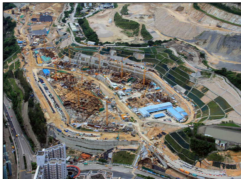
LR10 On-going Development Area at (DAR)
