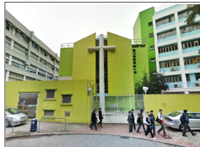
GIC1.10 SCHOOL AND INSTITUTE ALONG HIU YUK PATH AND KWUN TONG GOVERNMENT PRIMARY SCHOOL
