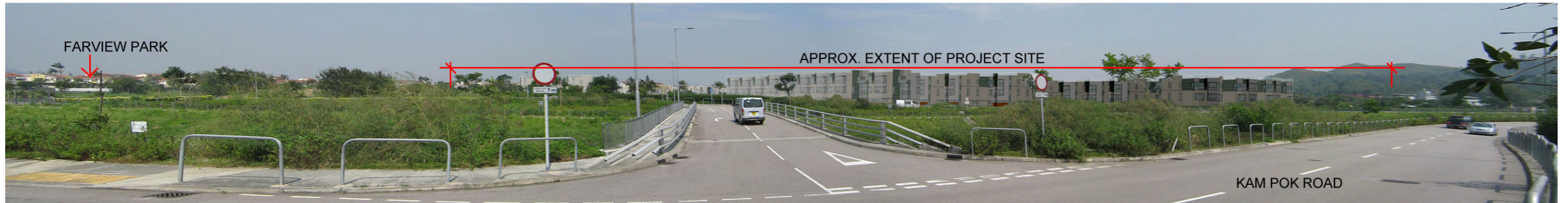
VIEW FROM VSR T1 BRIDGE ACROSS NGAU TAM MEI CHANNEL - DAY 1 WITHOUT MITIGATION (VIEW POINT 14)
