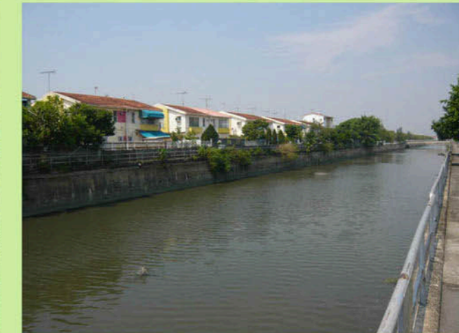
Nullah through Fairview Park
