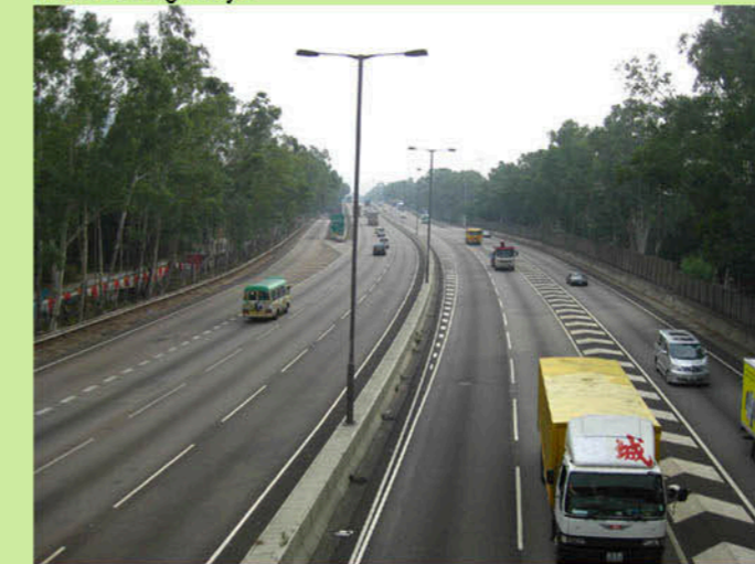
San Tin Highway
