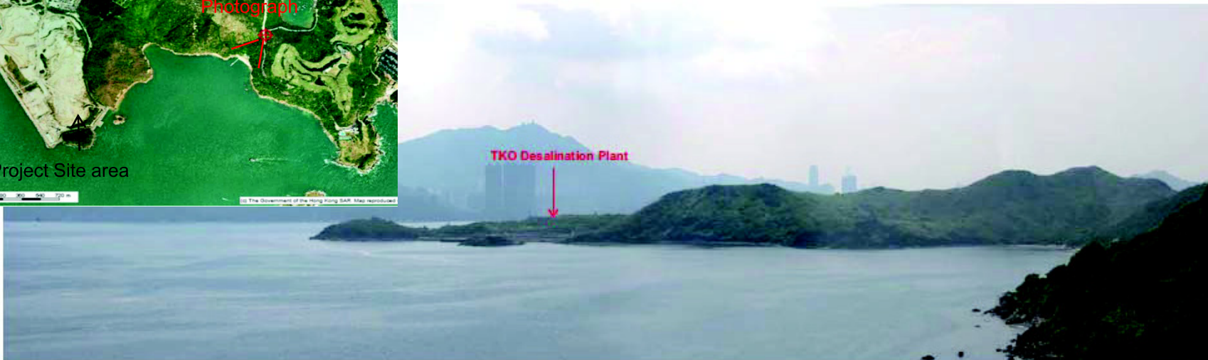
View towards the Project Site from elevated level of Tai Au Mun Road, near VSR R2 Clear Water Bay Golf and Country Club
