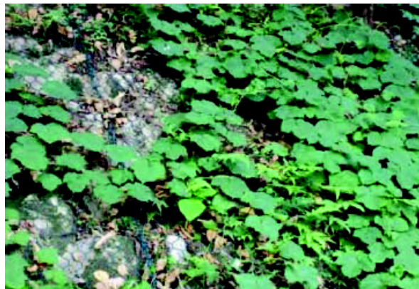
Undergrowth through wire mesh
