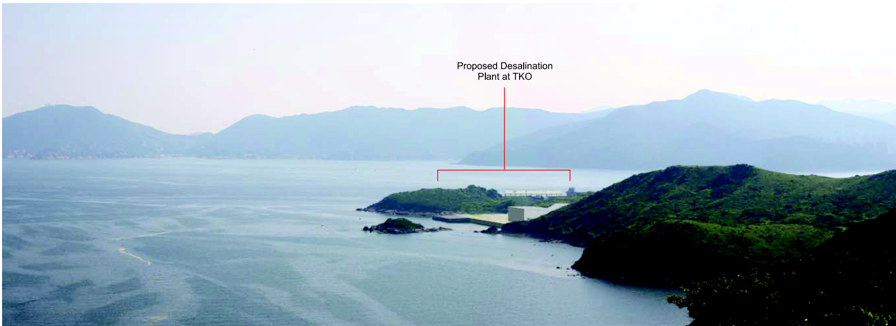
VP1 - View from High Junk Peak in Clear Water Bay Country Park on day 1 operation (without mitigation)
