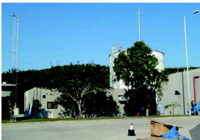
LR10 Site Office area of SENT Landfill
