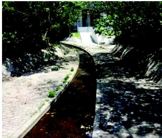
LR7 Drainage Channel
