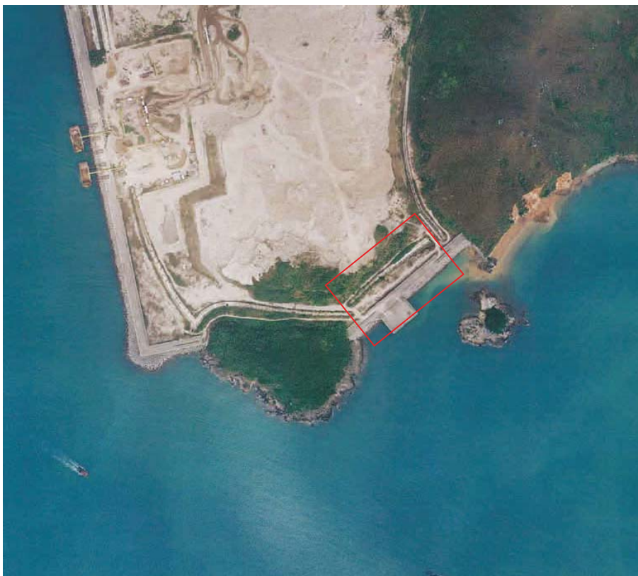
Year 2005 (ref: CW66157, height: 4,000ft) — No change of land use was observed compared to 2000. The TMS Site was left vacant and vegetation was observed growing within the Site. No activity was observed being conducted within the TMS Site.
