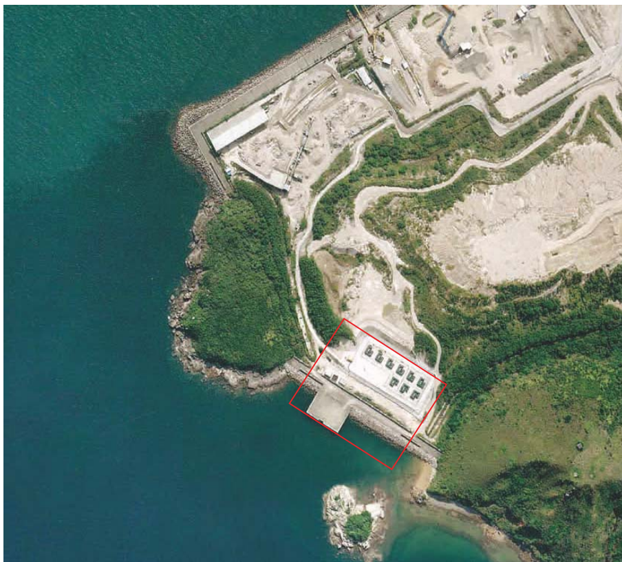
Year 2012 (ref: CS36650, height: 6,000ft) - The temporary magazine storages were constructed in 2012. Concrete pavement was observed within the TMS Site, except part of the access roads.
