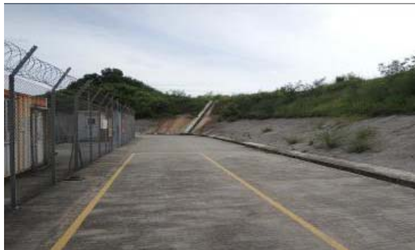
Concrete paved vehicle access road surrounding the magazine storages.
