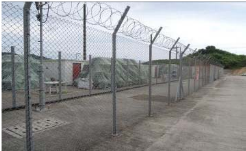
One of the magazine storages (with red door) surrounded by sand bags covered in tarpaulin sheets and fenced off from access.
