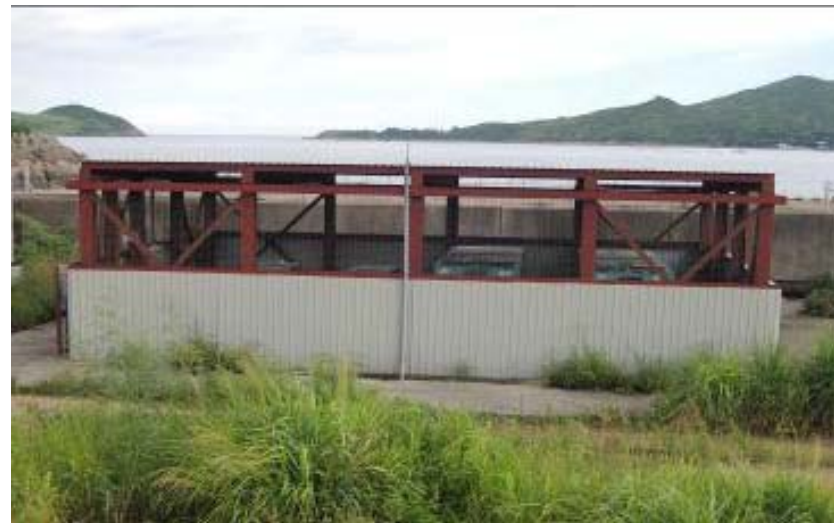
Generator Room surrounded and covered by corrugated metal
