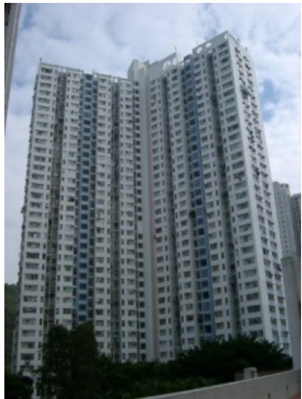
PYH1– Po Lam Estate - Po Yan House
