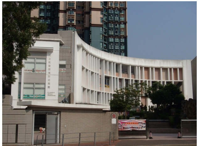
SACK1 - St. Andrew's Catholic Kindergarten
