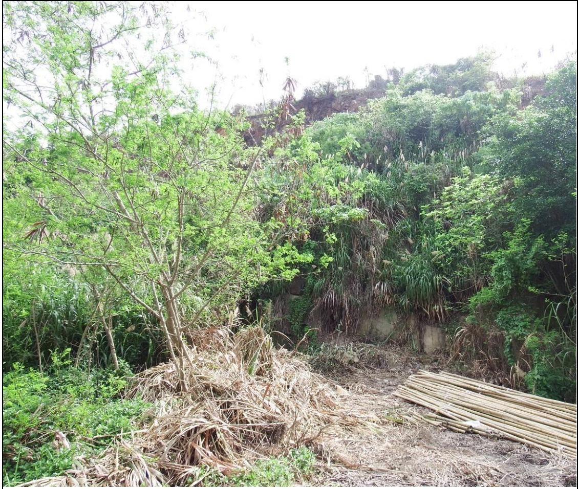
Plate 2: General view of study area for slope mitigation works
