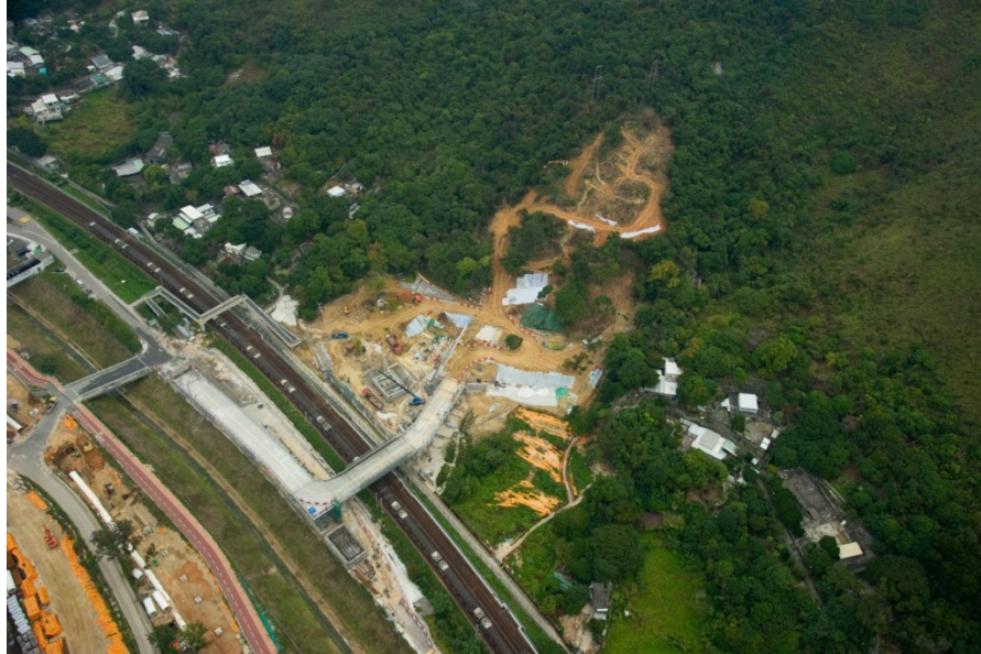
Figure 2.6 Site Photo of the Temporary Vehicular Bridge
