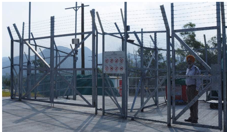
From top to bottom: A typical contractor's explosives vehicle; warning displays of loaded explosives vehicle; and a typical Magazine site.
