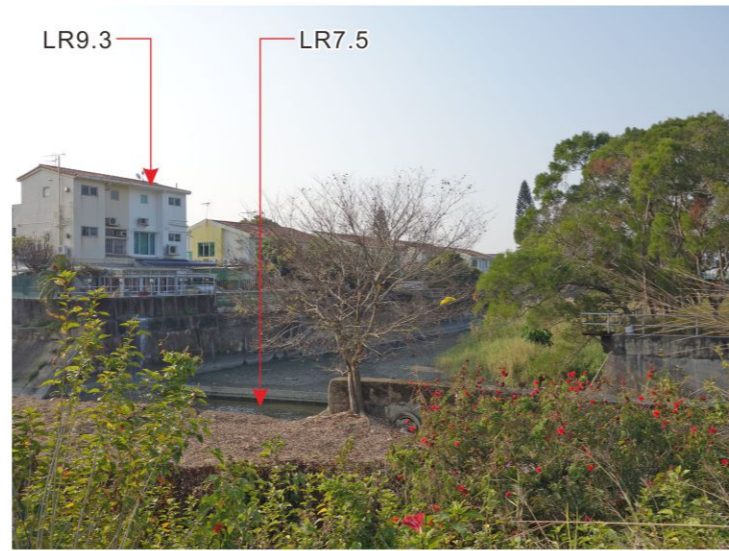
LR7.5 Fairview Park Engineered Water Channel
