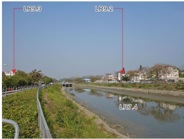
LR7.4 Ngau Tam Mei Engineering Water Channel
