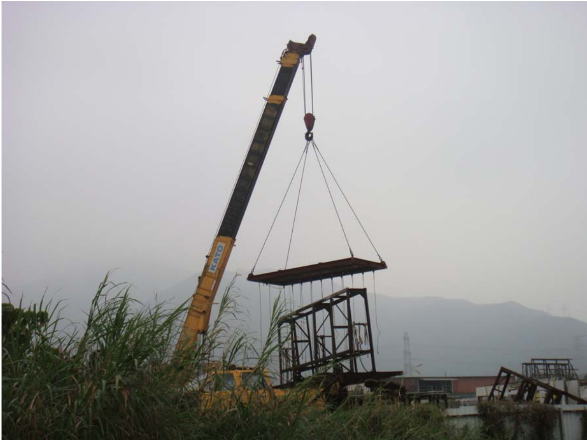
Plate 1: Mobile Crane at Open Storage (Fan Keung Kee)
