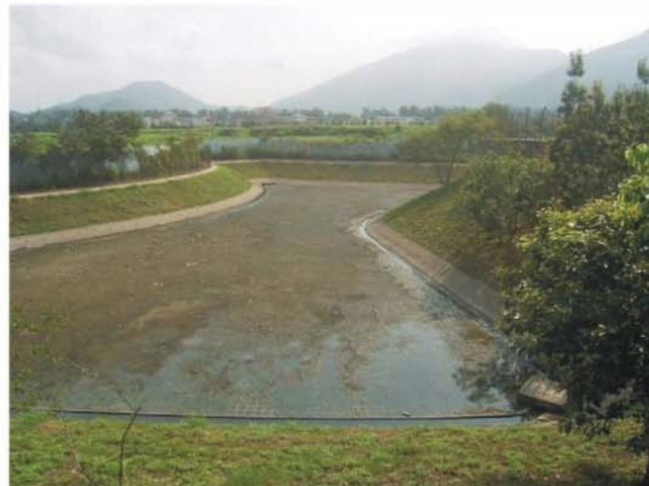
pond (flood storage pond)
