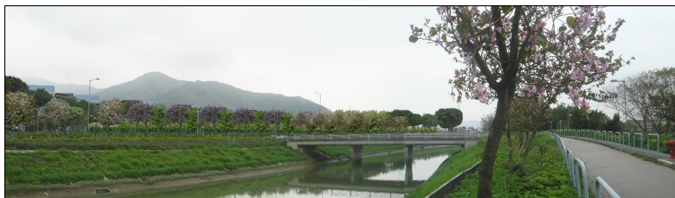
Figure 6.7: Restoration of perimeter planting
