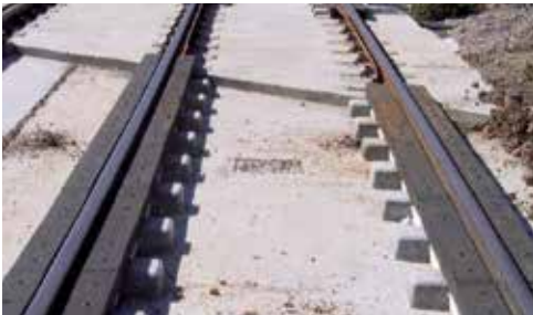
Concreted track with green track chamber elements and level crossing
