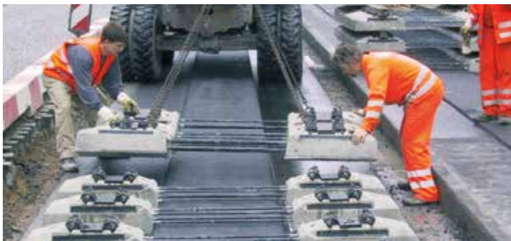
Placing the sleepers on the completed asphalt supporting layer
