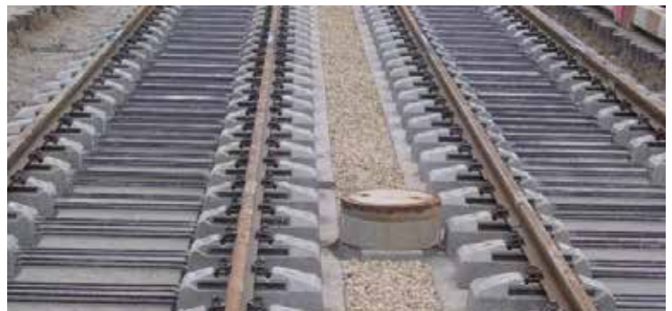
Installed and properly aligned track panels
