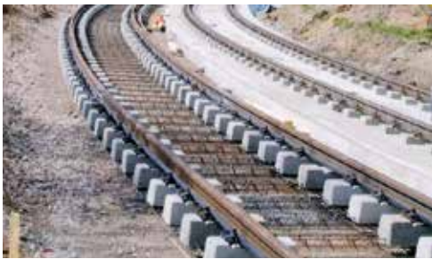
Completely assembled and aligned track panels
