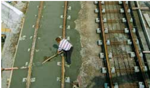
Concreting of the track panels
