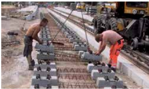
Positioning of the bi-block sleepers
