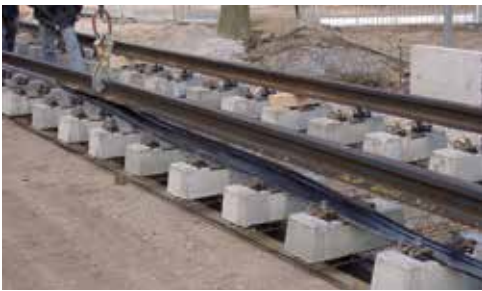
Attachment of the rail-flange sheathing
