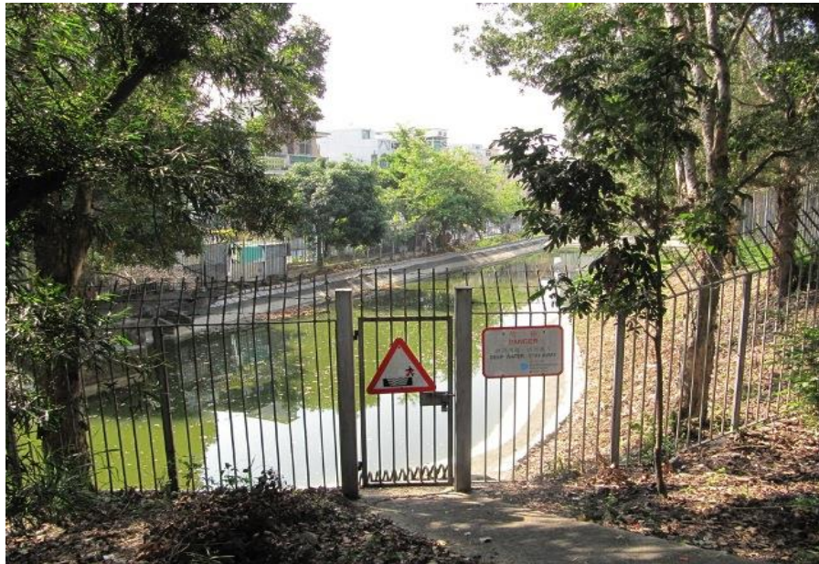
Storm Water Drain/Recreational Pond
