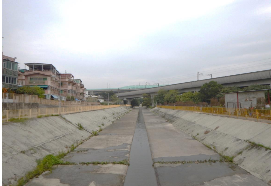
Modified Watercourse (Drainage) at Tsing Chuen Wai
