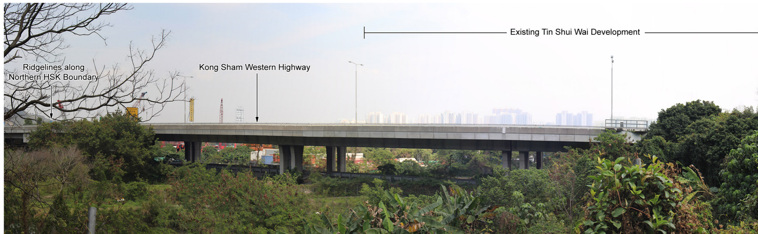
Existing Baseline Conditions
